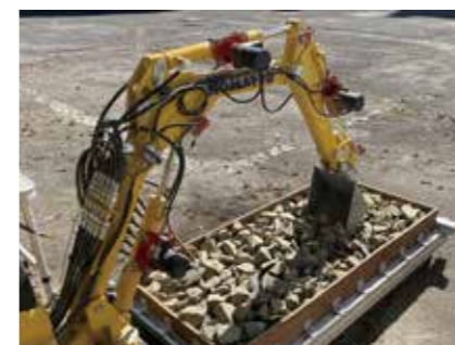
Fig. 4 Blasted-rock excavation by micro excavator
