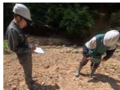
Fig. 3 Cone penetration test at actual river channel blockage site
