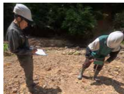
Fig. 3 Cone penetration test at actual river channel blockage site
