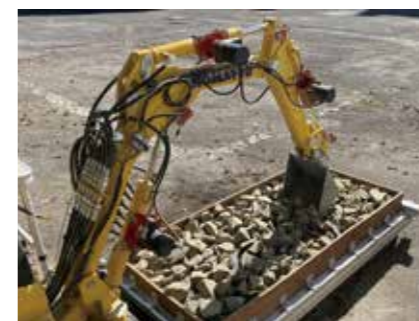
Fig. 4 Blasted-rock excavation by micro excavator
