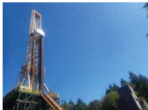
Fig. 1 Drilling site of geothermal field
