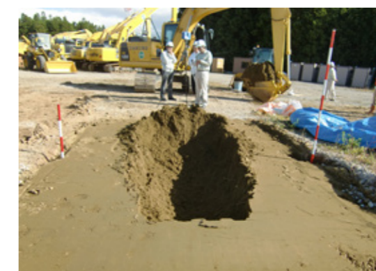
Fig.5 Excavation experiment using actual power shovel
