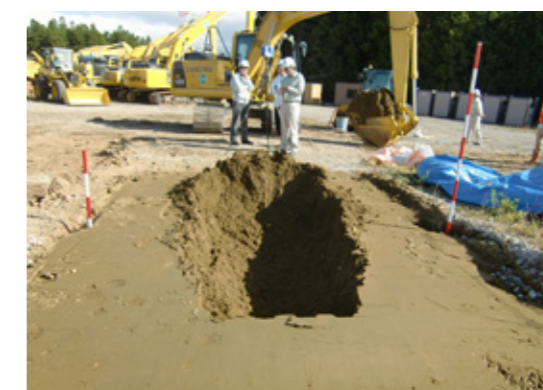
Fig.5 Excavation experiment using actual power shovel
