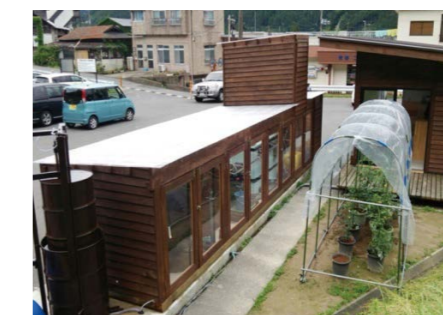
Fig.6 The compact & high efficiency methane fermentation system ( Yumeguri parking place in Naruko hot spring )
