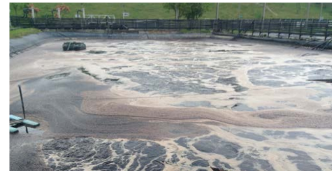
Aeration pond of a controlled landfill site in Southeast Asia.
