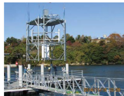
Fig.4 The tidal energy converter was installed by a crane ship (Sabusawa channel in Urato Archipelagos)
