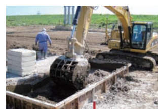
Fig.2 The actual construction to create the artificial ground by recycling Tsunami sludge.
