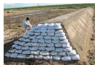
Fig.3 Artificial ground was completed.
