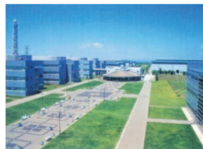
Fig.1 Nippon Steel R&E Center located in Futtsu, Chiba.
