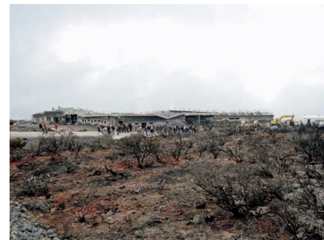
Fig. 4. New observatory under construction in Reunion Island.
