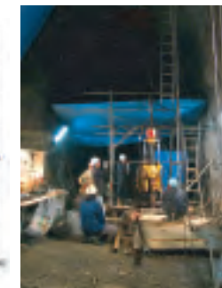
In-situ stress measurement by means of DCCBO technique.
