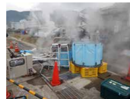
Fig.4 Field test of mechanical descaling.
