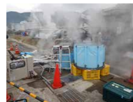
Fig.4 Field test of mechanical descaling.
