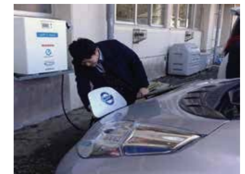
Fig.4 V2H system has been installed in Kazuma elementary school, Ishinomaki city (Task 3)
