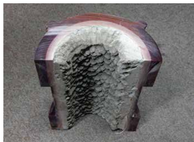
Fig.2 Pipe with Talc scale 3 month elapsed.
