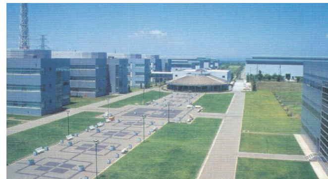
Fig.1 Nippon Steel & Sumitomo Metal R&E Center located In Futtsu, Chiba.
