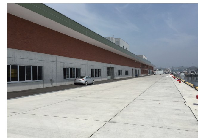
Fig.4 Onahama fish market which was built as reconstruction contracts from the Great East Japan Earthquake Disaster
