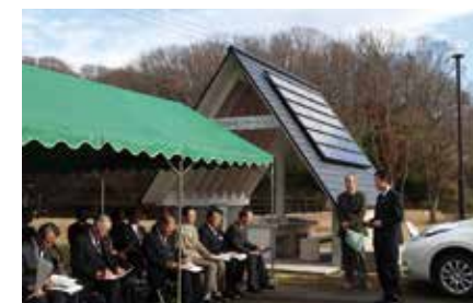
Fig.5 The installation ceremony of the Multi-Purpose Power Feeding Station in Osaki city(Task 3-a)
