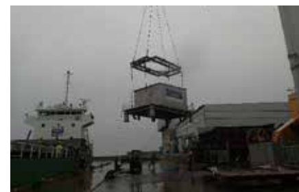
Fig.4 The unloading device from a ship at Kuji factory of Hitach Zosen Corporation (Task1 / Wave power generation)
