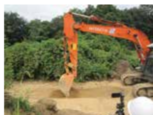
Fig.3 Soil excavation test by hydraulic power shovel with different soil strength characteristics and different bucket angle
