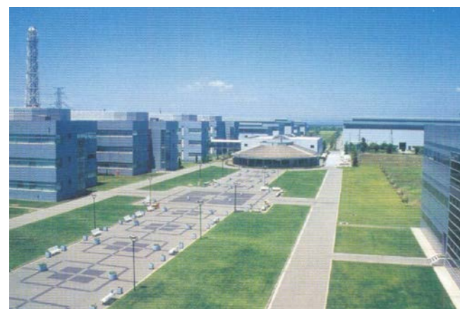
Fig.1 Nippon Steel & Sumitomo Metal R&E Center located in Futtsu, Chiba.
