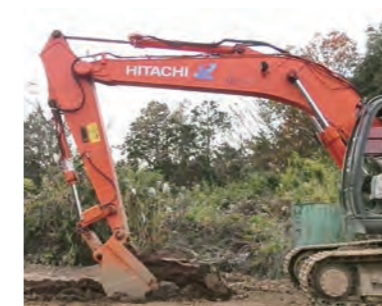
Fig.6 Soil excavation test using hydraulic power shovel
