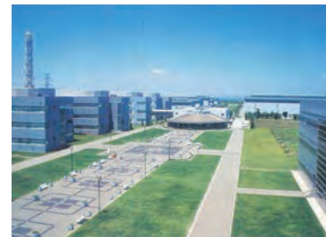
Fig. 1 Nippon Steel & Sumitomo Metal R&E Center located in Futtsu, Chiba.
