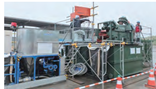
Fig.3 Screening and turbid water treatment system used in the trial construction
