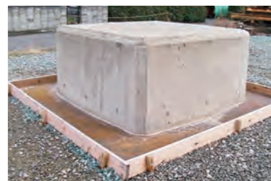
Fig.2 Embankment made by placing fiber-cement stabilized soil method
