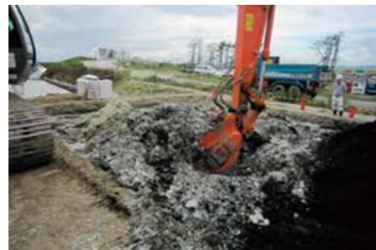
Fig.3 Actual construction to recycle Tsunami sludge in Natori city, Miyagi Prefecture
