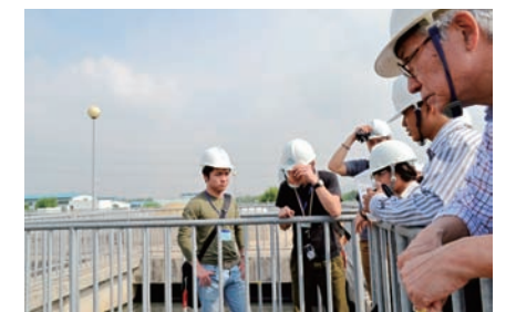
Fig.06 Binh Hung Waste Water Treatment, Vietnam
