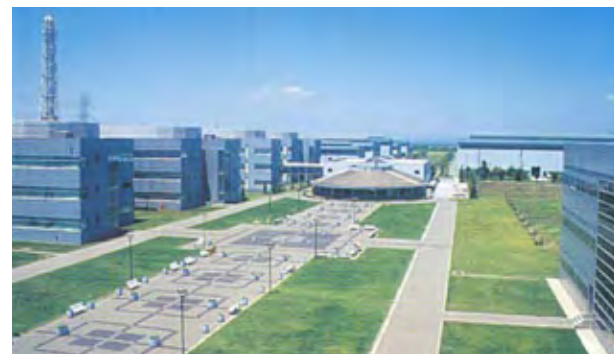
Fig.1 Nippon Steel R&E Center located in Futtsu, Chiba.
