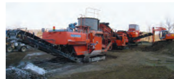
Soil modification using two mobile modification machines. Waste gypsum powder is added to soil in first machine and lime is added in second machine.
