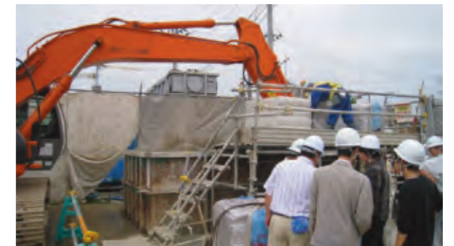
Visit to a site of tunnel excavation for the Sendai city subway (Yakushi-do area): At this area, the sludge discharged during the ground modification is recycled by the fiber-cement-stabilized method. All of the modified soil is used as road embankment material at Akiu area.
