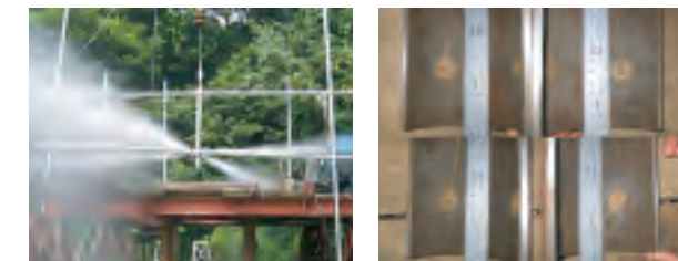
Multiple nozzle system for perforation at field.
