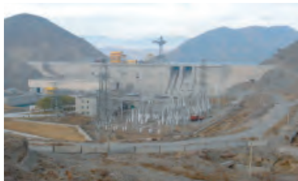
Hydraulic power plant over the Naryn River (headwaters of Syr Darya river) in Kyrgyz Republic: one of the causes of water war in Central Asia
